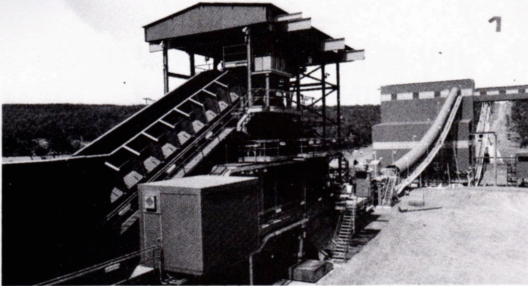
(MOBILE PRIMARY CRUSHER AND MINESITE CONVEYOR, MOUNT SADDLEBACK, WESTERN AUSTRALIA)
